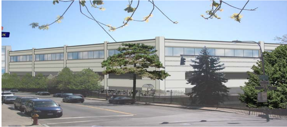
Rendering of the proposed development from the corner of Warburton and Ashburton Avenues.
